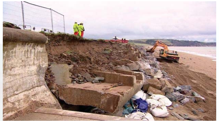
Collapse of the seawall at Torcross
