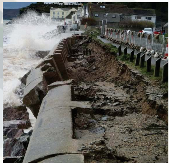
Collapse of the seawall at Torcross
