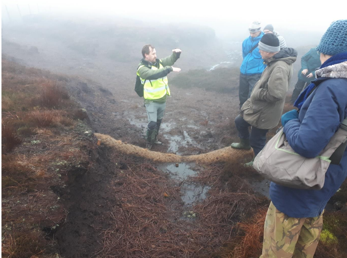
Figure 1: Coir rolls used to block gullies in upland raised peat bog.
